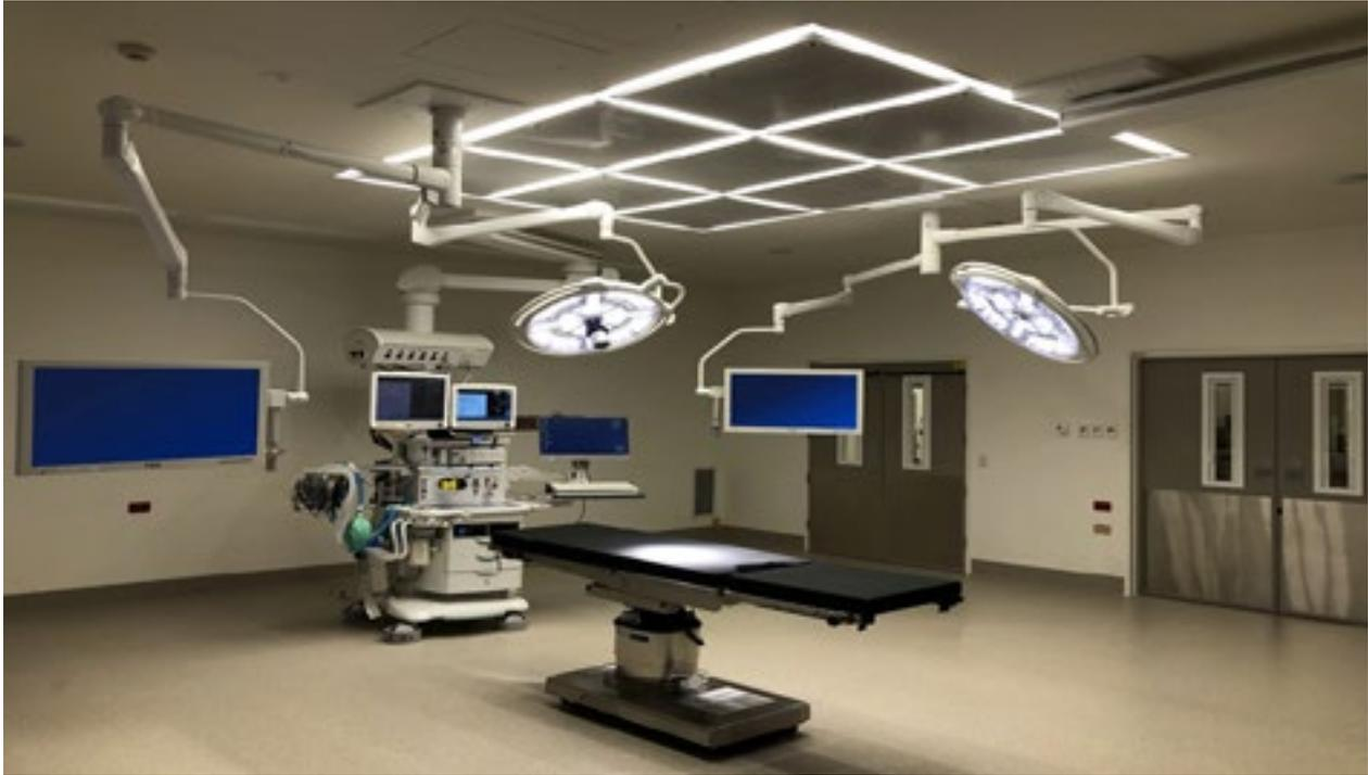
*Illustration 4: Modular, single large diffuser system with light and boom mounts placed outside of the array. Includes integral, engineered lighting system that helps to reduce turbulence. (Source: Wilhelm Integrated Solutions)*
